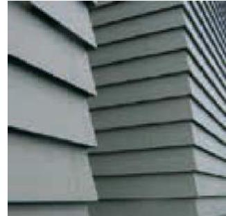
For single top edge or bottom edge fixing the panel should be no wider than 300mm. Any wider than this and the panel should be both top and bottom fixed.
