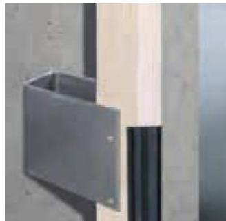
The U-connector is secured to the wall with suitable anchors. The same principle remains when using metal, always place a thermostop between the metal and the backing wall.
