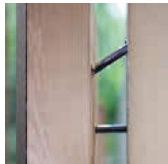
The recommended centres and arrangement for the structural distance screws is per screw manufacturer’s details. The distance screws are arranged in a horizontal and angled arrangement. The horizontal screws maintain the distance to the wall while the angle screws prevent the supporting frame from slipping.
